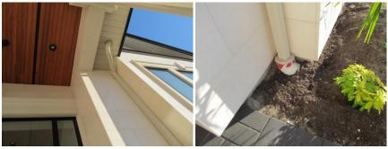
★ The top level downspout is suggested to extend to lower gutter to avoid roof shingle pre-mature damage.(建议将上层下水管延伸至下层檐沟)
