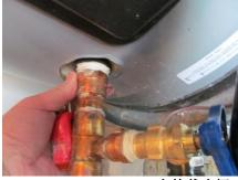
Water Shut-Off Valve (水的截止阀)
