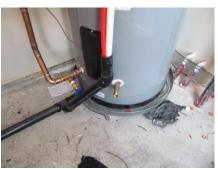
Seismic Straps (防震加固)
