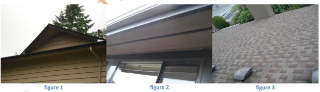
convection that caused the heat conducted and lose even without vents installed; most important although there is a vapour barrier under the attic insulation, the air can always find its way to get into attic. It would condensate if not vented for the lower temperature in the attic. This would cause the mould and mildew, even rot structure. In the long time, it would not only be a comfort issue but a safety hazard.
