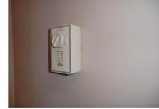
Some baths should have the fans running occasionally and 5-10 mins after shower if there is no window. In the newer buildings the humidistat has been installed, which is automatically controlling the fan in hallway bath. We recommend setting it at 50-60% in summer & 40-50% in winter
