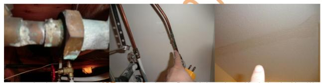
the same time because the metal resources kept going up, Pex took the major position in the plumbing. We normally do not have too much worry on Pex pipes during inspection. However, recently CBC exposed the negative news on Pex blast, which is involved in the Kitec made from 1995 to 2007 mostly orange yellow and blue color. This taught us that nothing is 100%. The actual observation & experience are the objective judgement
