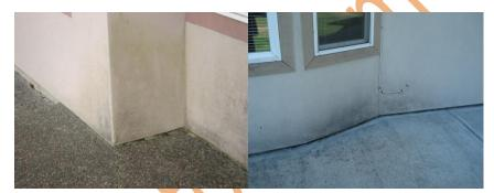
The most condition of conventional stucco wall is the crack. It normally showed up in my inspections, which is most often located at the sides of doors or windows, the corner of walls. This is caused by the stress
